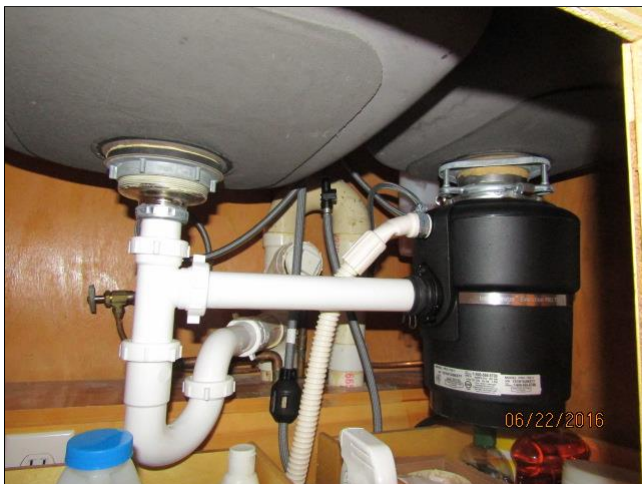
B. Item 2(Picture) Kitchen Sink Drain lines.
