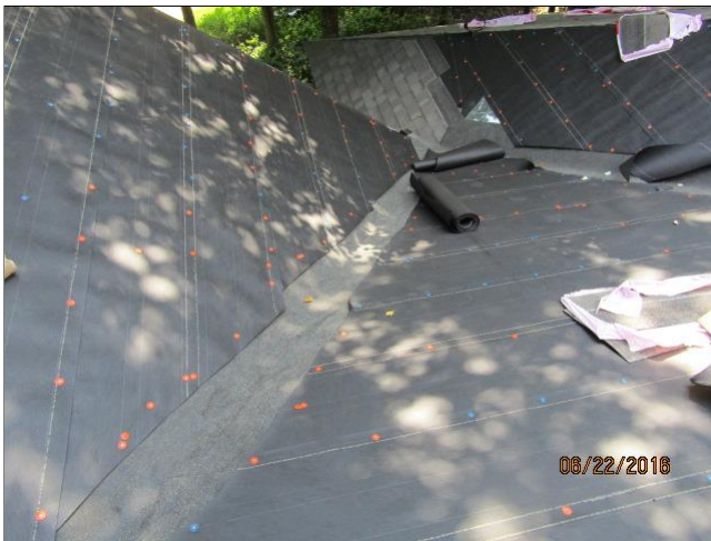
C. Item 3(Picture) Sufficient valley flashing.
